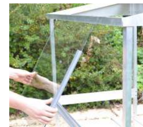
A. Fitting the glass
