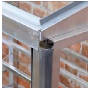
Corner trim in place
