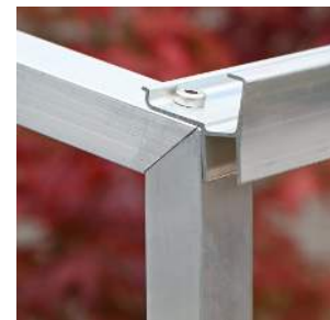
IMAGE 4 No gap in mitre and front top rail fitted properly
