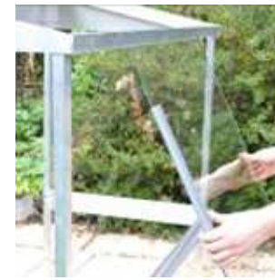
C. Fitting the glass
