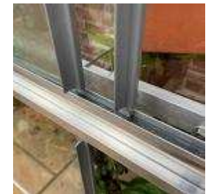
Glass in channel with two sheets overlapping
