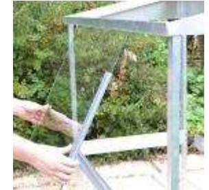
A. Fitting the glass
