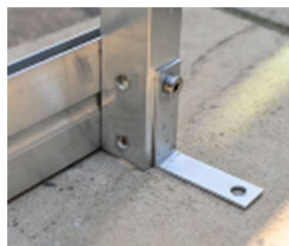
ANCHORAGE BRACKET FITTED
