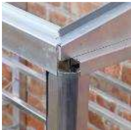
Corner trim in place
