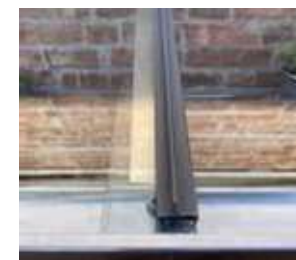
Roof glass overlapping
