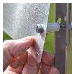
Nylon spacers on infill plate
