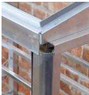
Corner trim in place
