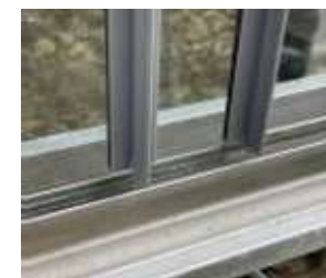
Glass in channel with two sheets overlapping
