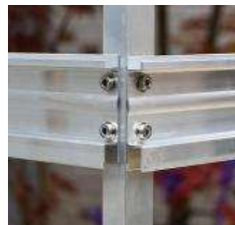
THE DEEPER CHANNEL GOES AT THE BOTTOM
