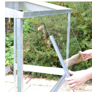
C. Fitting the glass
