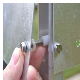
Nylon spacers on infill plate
