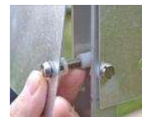
Nylon spacers on infill plate
