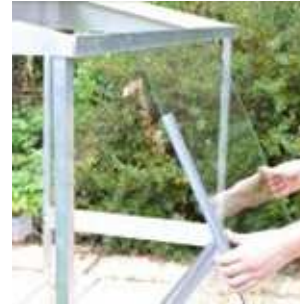
C. Fitting the glass
