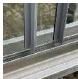
Glass in channel with two sheets overlapping
