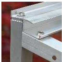
FIXING DETAIL
