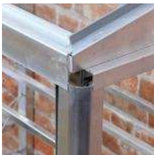
Corner trim in place
