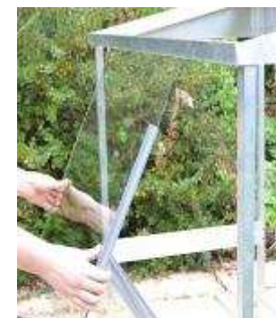
A. Fitting the glass
