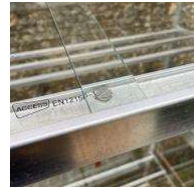
Roof glass overlapping
