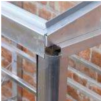
Corner trim in place
