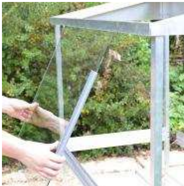
A. Fitting the glass
