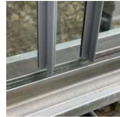
Glass in channel with two sheets overlapping
