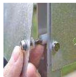
Nylon spacers on infill plate
