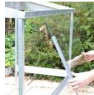
C. Fitting the glass
