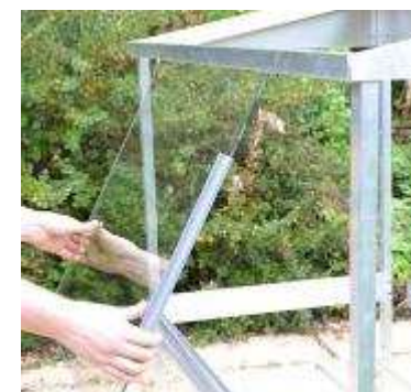
A. Fitting the glass
