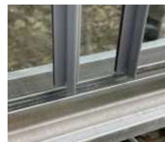
Glass in channel with two sheets overlapping
