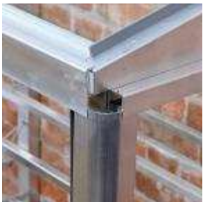
Corner trim in place
