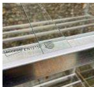
Roof glass overlapping
