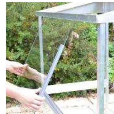
A. Fitting the glass
