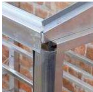
Corner trim in place
