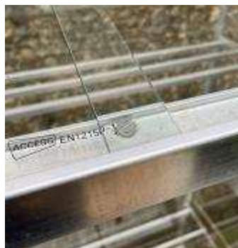
Roof glass overlapping
