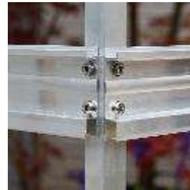
THE DEEPER CHANNEL GOES AT THE BOTTOM
